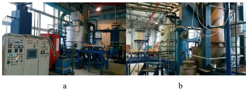
Fig. 5. Technological line for hazardous waste processing: control panel (a), the system of gasification products cleaning (b)
